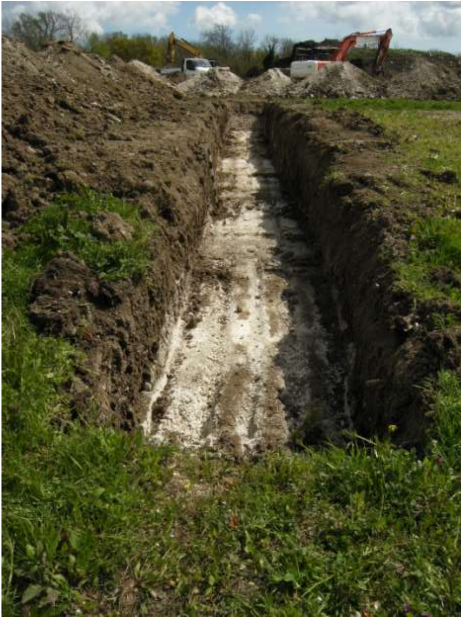
Plate 16. Trench 9 looking southeast
