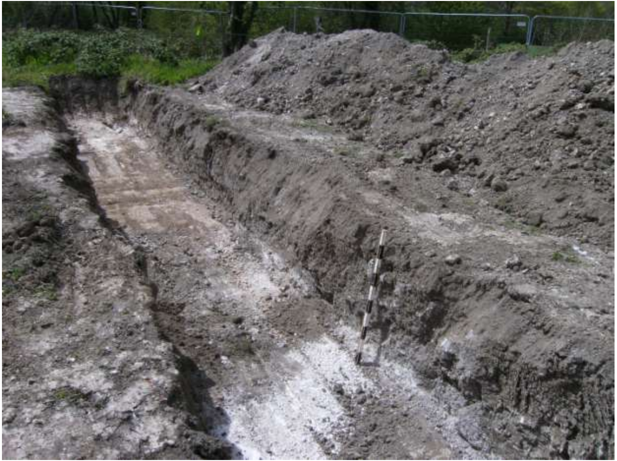
Plate 7. Trench 4 from the southeast, one-metre scale
